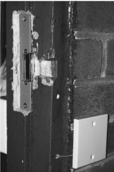
**Figure 10-17** The RFID antenna installed outside the door
